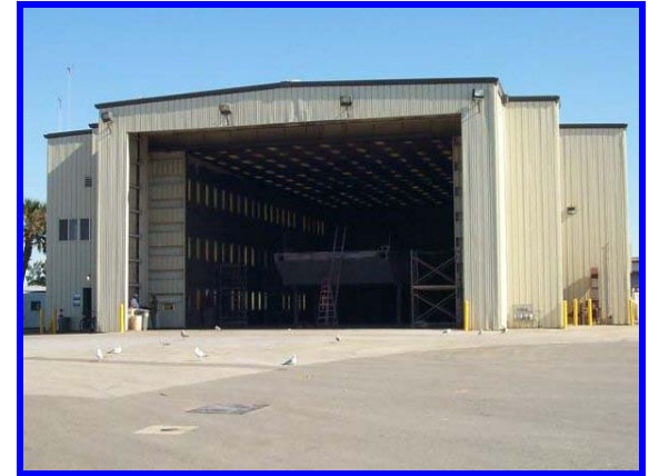
Environmentally Controlled Blasthouse for sections up to 120 tons
