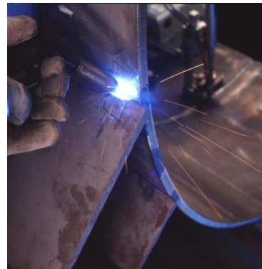
Shielded Metal Arc Welding
