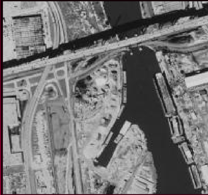
Aerial View Bollinger Gulf Repair LLC
