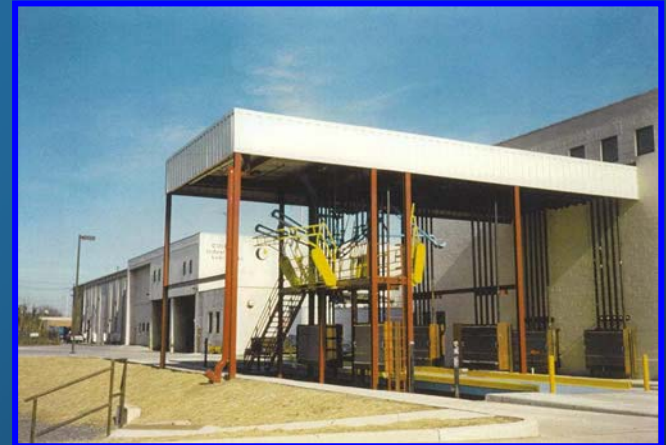
Loading/unloading rack area
